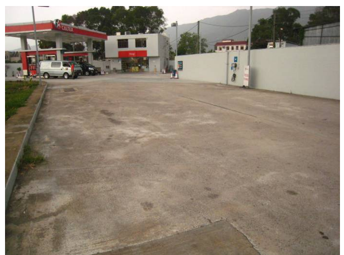
P6. Caltex Petrol Filling Station (PFS3) is concrete paved
