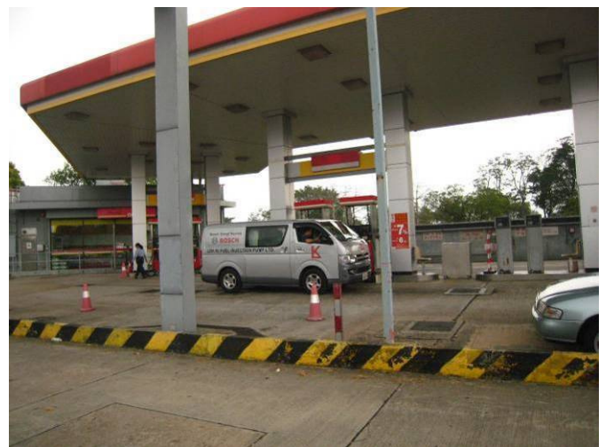
P4. Sinopec – Shek Kong Petrol Filling Station (PFS2) is concrete paved
