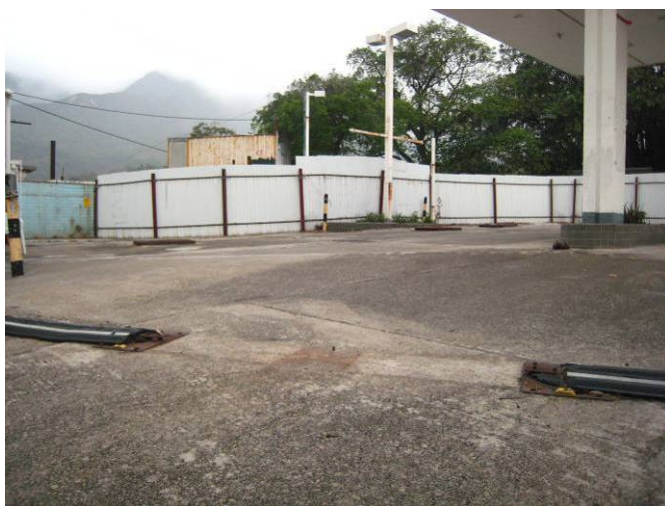
P9. Closed Petrol Filling Station (PFS5) is concrete paved
