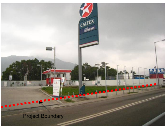
P5. Caltex Petrol Filling Station (PFS3) located outside the project boundary
